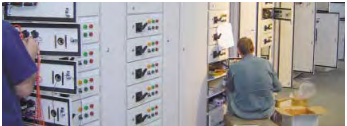
Motor control centre under construction
